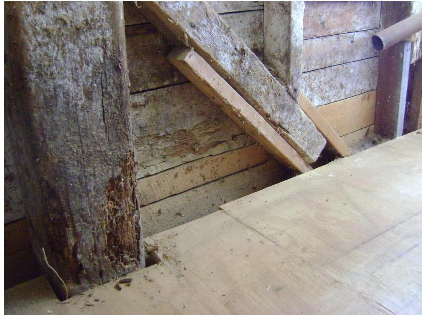
*Photo #8 - Repairs indicating possible decay at sills from animal wastes.*
