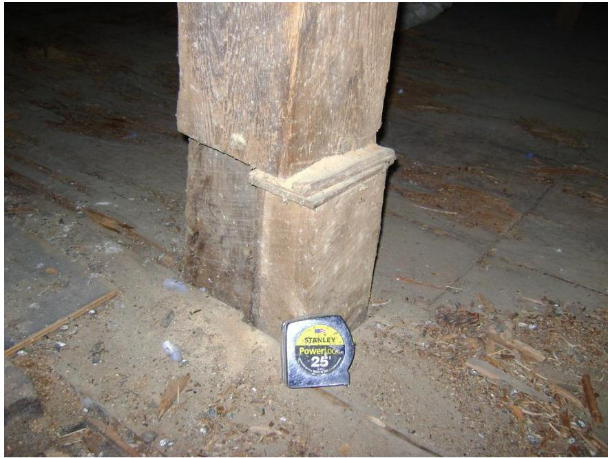
*Photo #10 - Post 3C, cut off and shimmed, also active insect boreholes and frass evident.*
