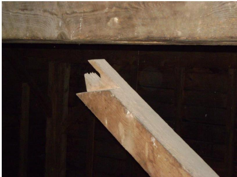
*Photo #12 - Disconnected knee-brace, indication of settling and distortion of major frame timbers such as Post 3C.*
