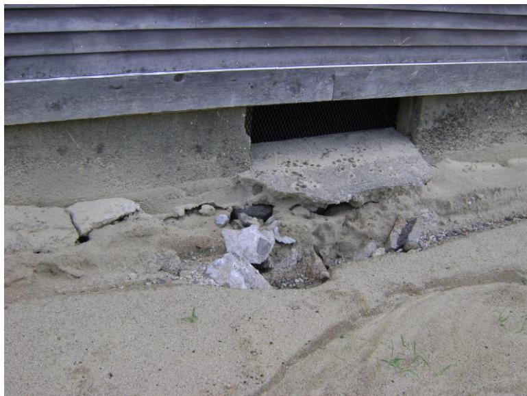
*Photo #6 - East foundation, water infiltration and soil erosion.*
