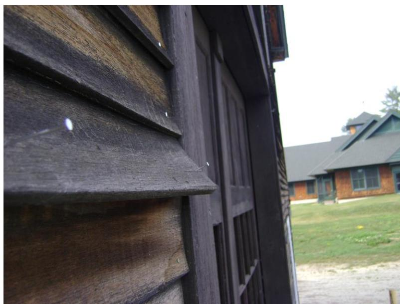
*Photo #18 - Clapboards warped and detached, with nails pulled. Typical of many.*
