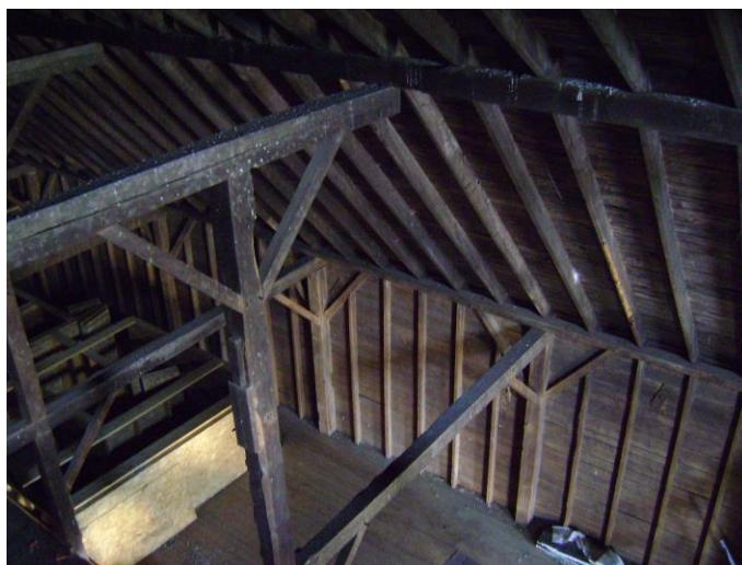
*Photo #2 - Typical view of barn frame showing heavy timber "bents" and "balloon" type wall studding.*
