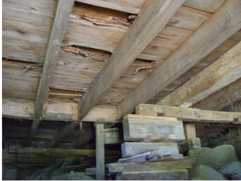
*Photo #7 - Northwest section of undercarriage, damage to floor and sub-floor framing, temporary cribbing.*
