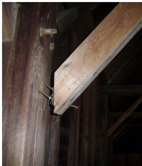
*Photo #13 - Nailed knee-brace connection at wall post separated. (Typical)*
