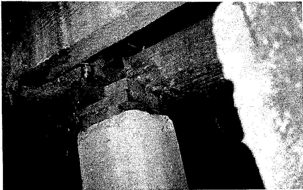
Damaged beam along 2 between C & D
