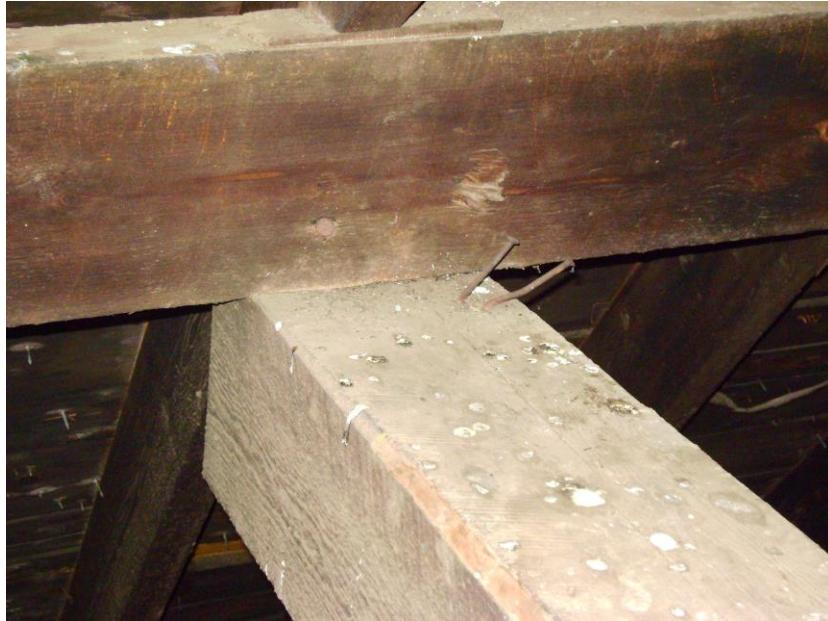
*Photo #14 - Structural major roof purlin attached to bent by toe-nails only.*
