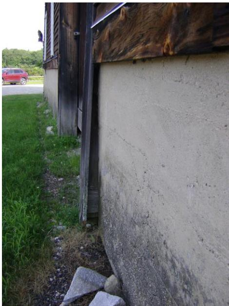
*Photo #5 – West foundation, concrete stem-walls leaning out at top.*
