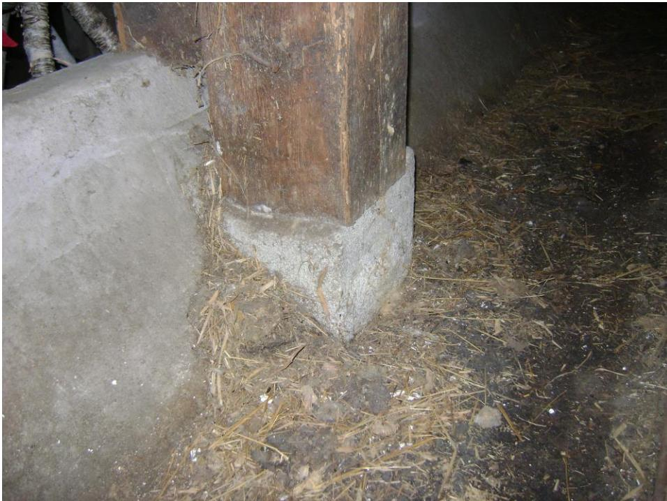
*Photo #9 - Concrete feed trough with step for shortened primary post. (Typical)*
