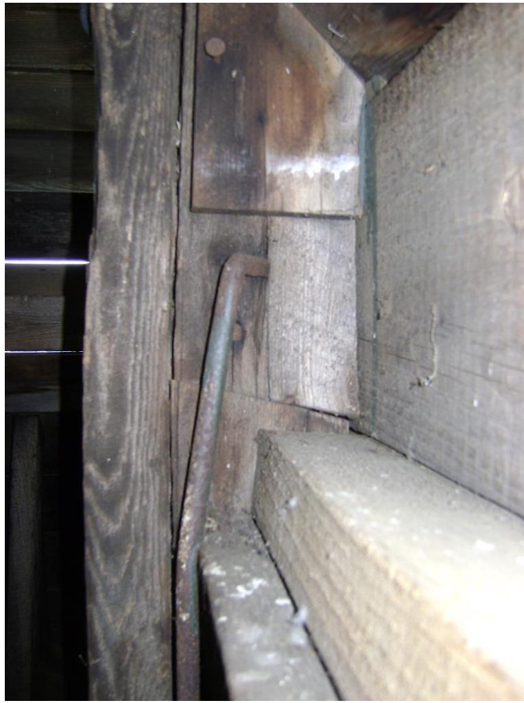
*Photo #21 - Interior of Cupola, showing iron staple anchoring cut post. (Typical)*
