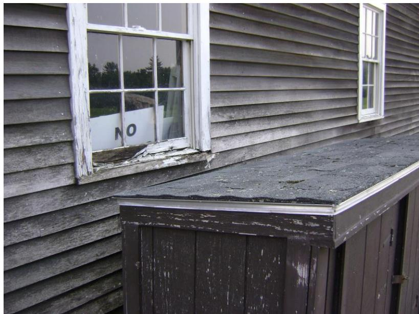
*Photo #19 - Water damage to window resulting from proximity of bin assembly.*
