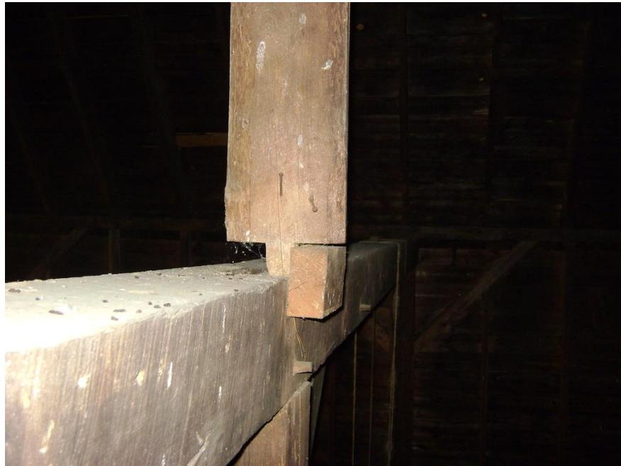
*Photo #11 - Displaced tenon at tie beam above post 3C. Vital roof support is potentially compromised.*
